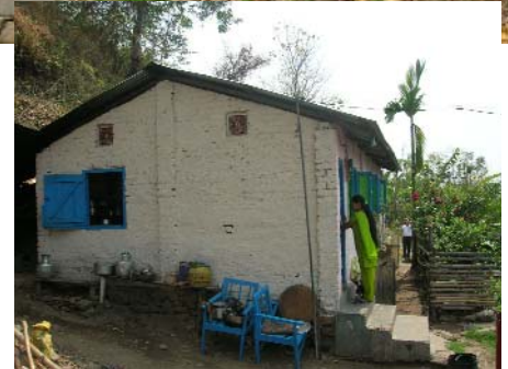
Front and the rear view of the church building at Dhudia
